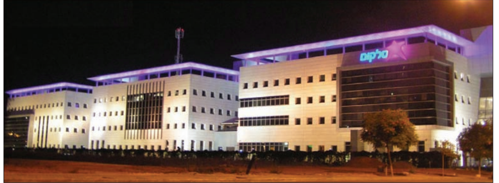
Cellcom Telecommunications, Inc. • Netanya, Israel
